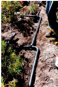
Figure 5: A branched drain graywater system, which relies on gravity (source: centralgraywater.org ).
